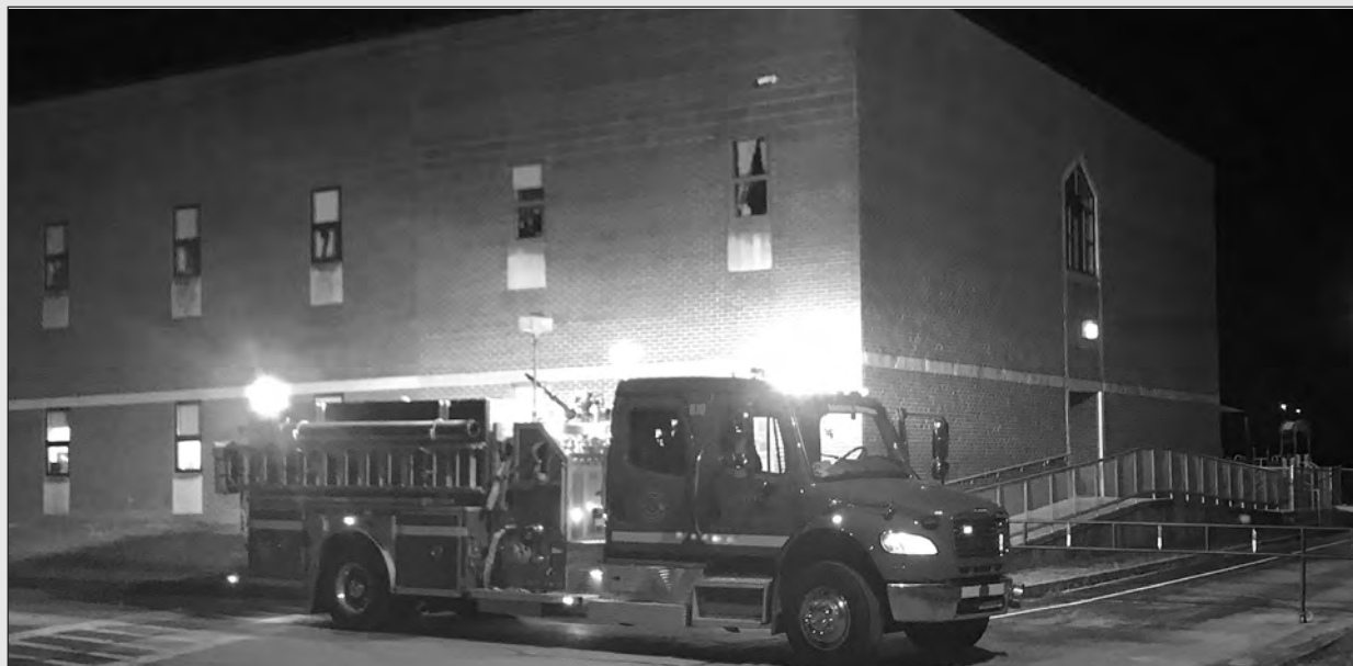
The Mount Vernon Fire Department was called to the Mount Vernon Elementary School Friday night after smoke was reported in the building. Once on the scene, first responders learned the smoke was from a faulty heating and cooling system and no fire had occurred. Fire fighters ventilated the building and no damage was reported from the smoke.
