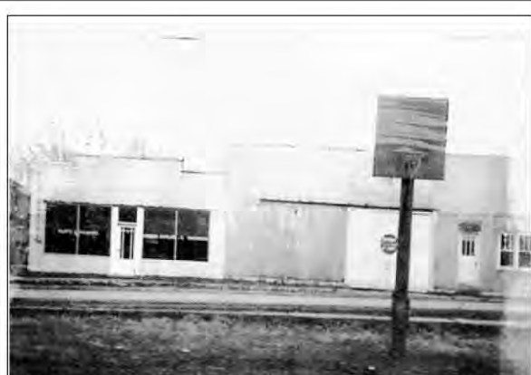
Building when it was first leased - 1971
