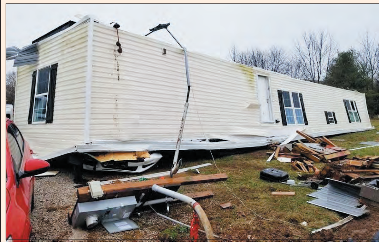
This mobile home was torn from its foundation and flipped over onto its top during Saturday's heavy storms in the Brindle Ridge area. Officials say the home rolled onto a car in the driveway and two occupants were inside the home when it rolled. However, neither occupant was injured. Reports of wind damage came from all areas of the county but no injuries were reported.
