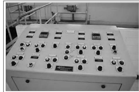
The water inside the building, at the Mt. Vernon Walter Plant, is constantly monitored by computers which perform tests making sure the filters stay clean. The monitors also let operators know when a filter needs to be removed and cleaned.
