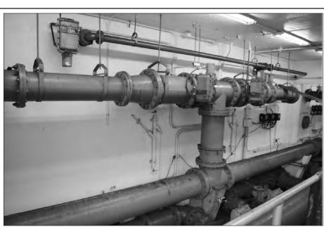
Water passes through large pipes inside the Mt. Vernon Water Plant, feeding it into filters that add polymers which causes algea molecules to stick together making them easier to filter out of the water.
