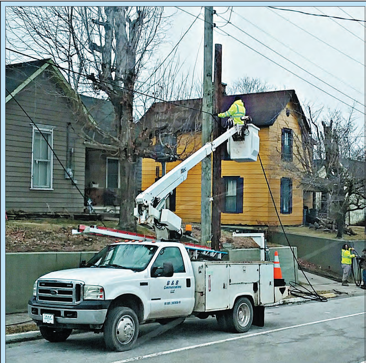
B&B Communications, out of Hazard, is busy installing TV cable in Livingston. According to Livingston Mayor Jason Medley, the company, which is already hooking up customers in Livingston, will eventually reach 200-300 customers in Livingston and surrounding areas.
