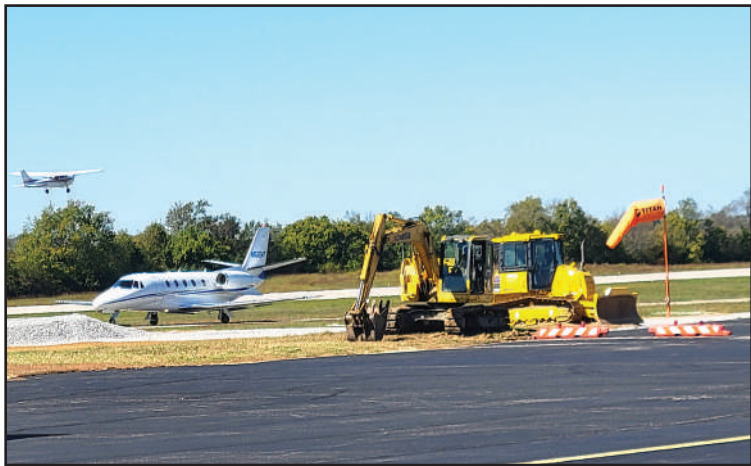
A water/sewer construction project to serve the Central Kentucky Regional Airport is encountering a potential delay, while work on a $3 million terminal building is expected to begin next year. The terminal is just one of the construction projects underway at the airport.
