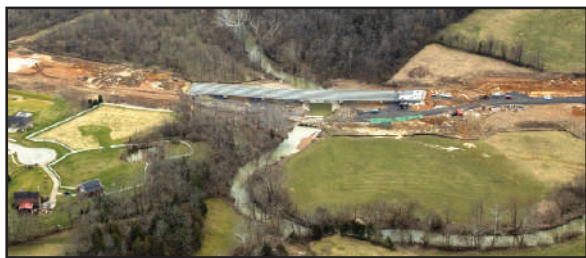
An aerial photo shows current construction of a bridge over Silver Creek recently. Photo by Mike Cyrus
