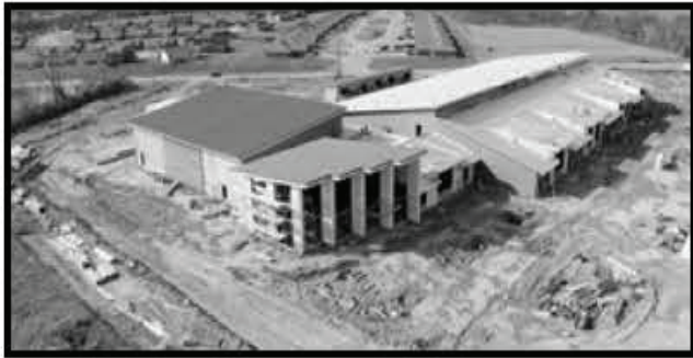
The Ignite North campus behind Toyota South in Richmond.
