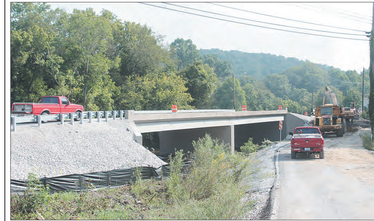
The Dix River Bridge at Brodhead was reopened to motorists last Friday. The bridge was originally condemned by Kentucky Transportation Cabinet engineers last November when, during a routine inspection, they realized the bridge's center box beam had severely decayed and posed an immediate threat to motorists. A temporary bridge was built in January and will now be torn out with large track excavators. A lot of the material from the temporary bridge will be recycled and used on other KYTC projects.
