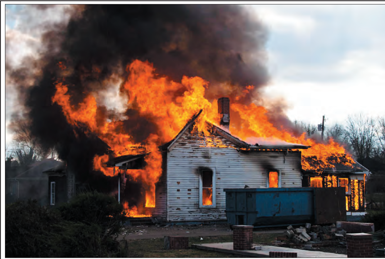
Brodhead Fire Department and Mt. Vernon Fire and Rescue responded to a house fire last Friday on Maple Street in Brodhead. Authorities say the abandoned house was owned by Brodhead Baptist Church, who was in the process of demolishing the house. Officials believe workers were burning debris next to the house when it caught fire. No one was injured in the fire.
