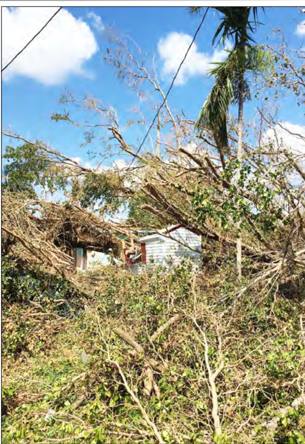
A Florida home is destroyed by trees after the hurricane. This picture was provided by Berea Municipal Utilities Director Ed Fortner, and was taken by one of the BMU workers who helped bring electricity back to thousands of customers.
