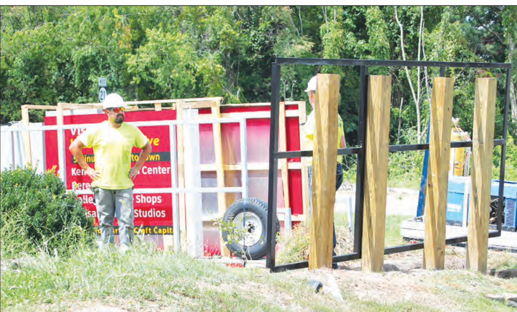
New signs have been showing up around Berea the past two weeks, as the culmination of the Wayfinding Project that Berea Tourism had started years ago. Above, workers install the Berea Sign on Highway 25, outside of Knight's Inn.
